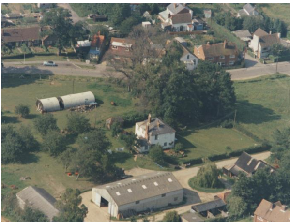
Court Farm House and farmyard - 1973?
